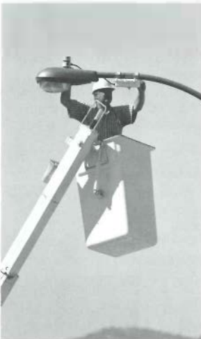
Installation of radio on light pole
