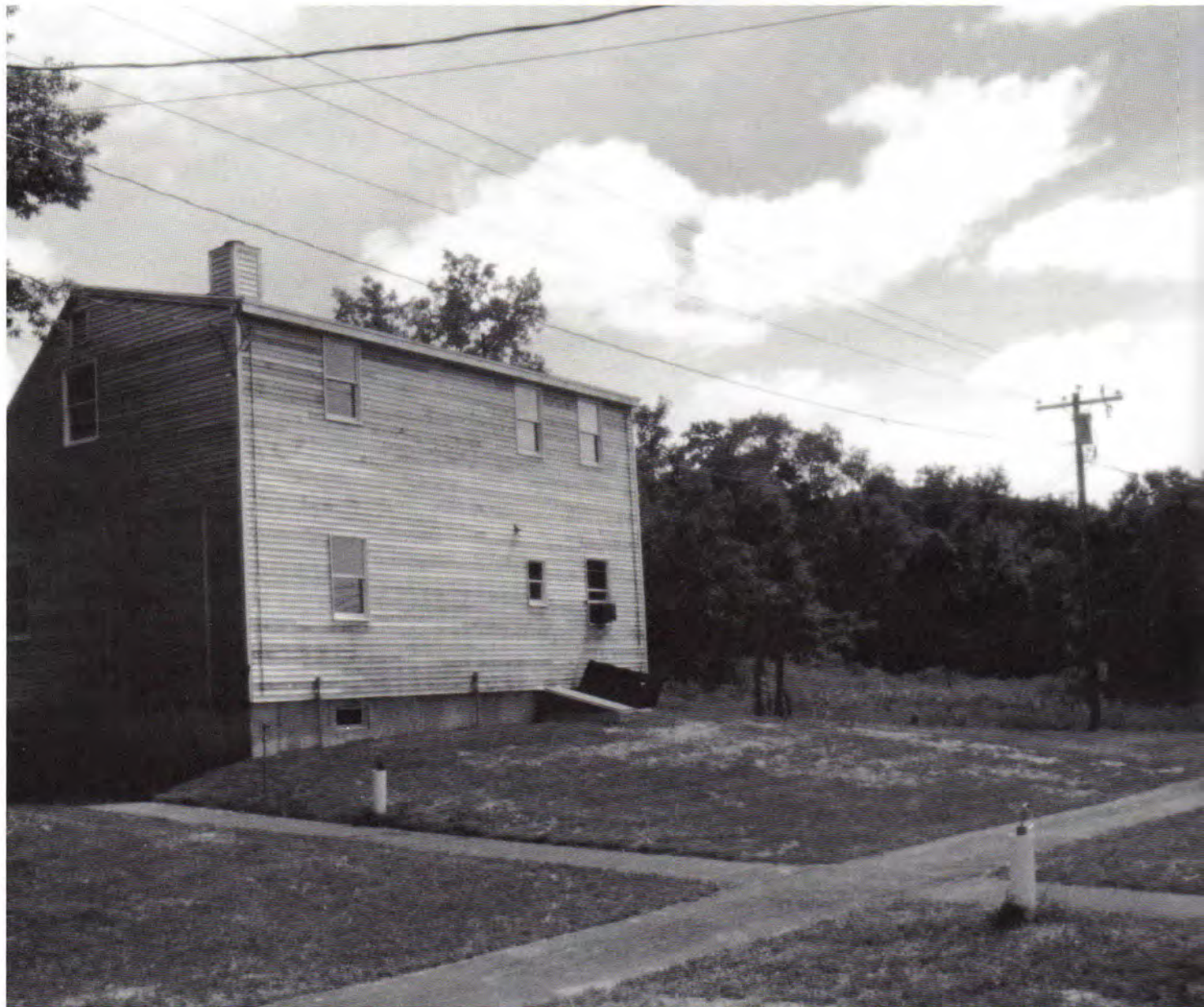
Laboratory house and overhead distribution line
