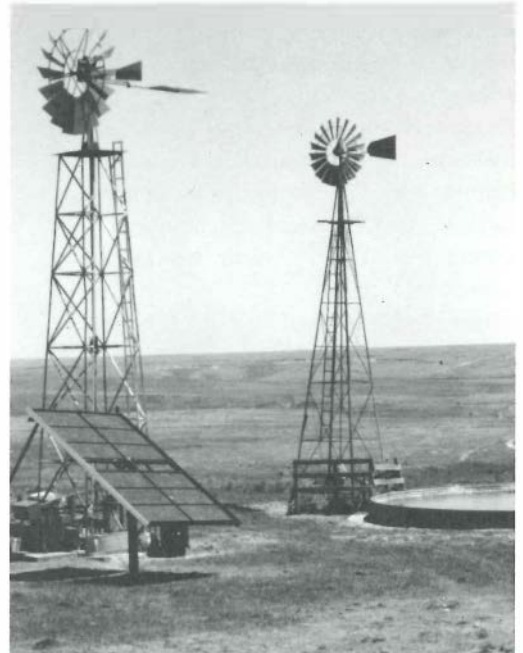
Livestock water pumping
