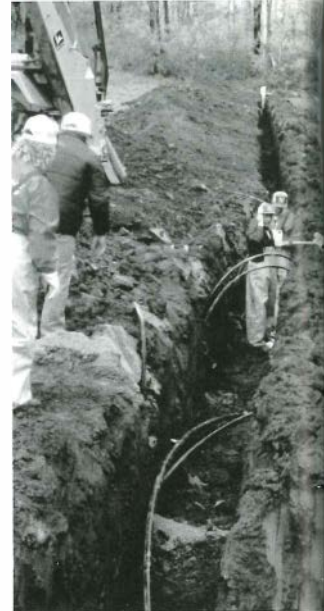
Installing horizontal ground loop
