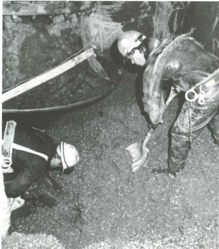
Removing mounds of mussels from a pump house
