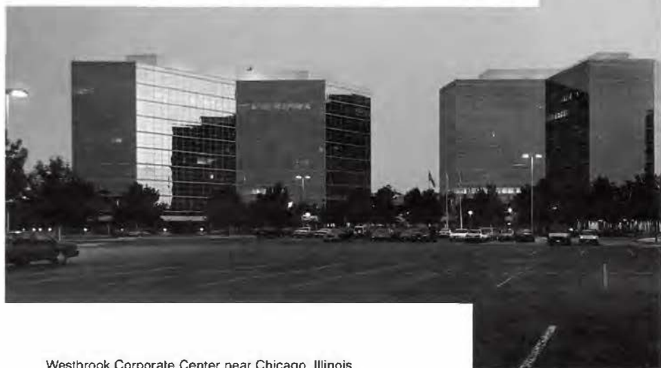
Westbrook Corporate Center near Chicago, Illinois
