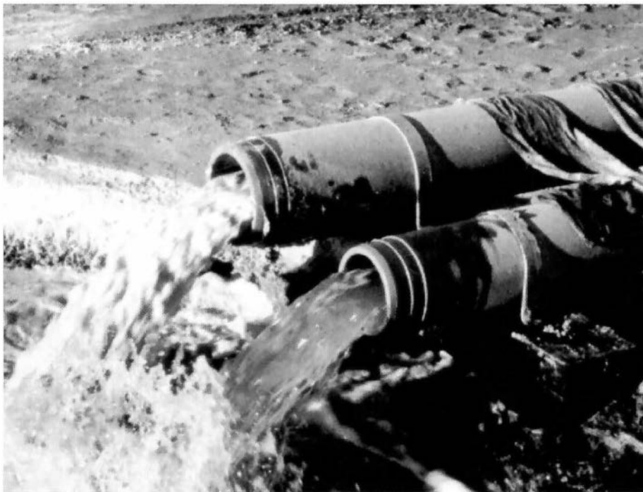
Figure 1 Codisposal of low-volume noncombustion wastes (bottom pipe) and high-volume combustion wastes in an ash pond. EPRI has gathered environmental data on this utility practice, called comanagement, for use in regulatory review.
