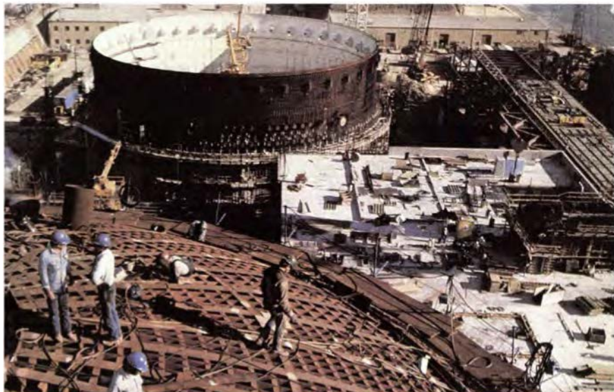
Nuclear plant construction
