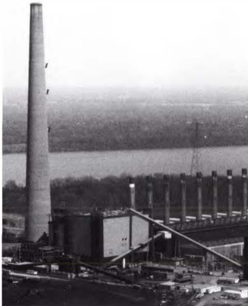
AFBC unit (left) at TVA's Shawnee plant
