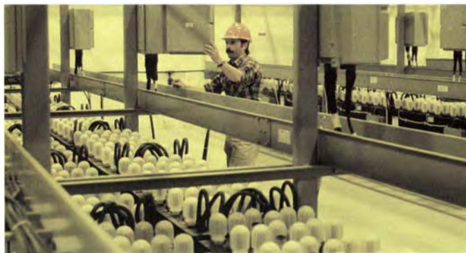
Battery Energy Storage Test Facility
