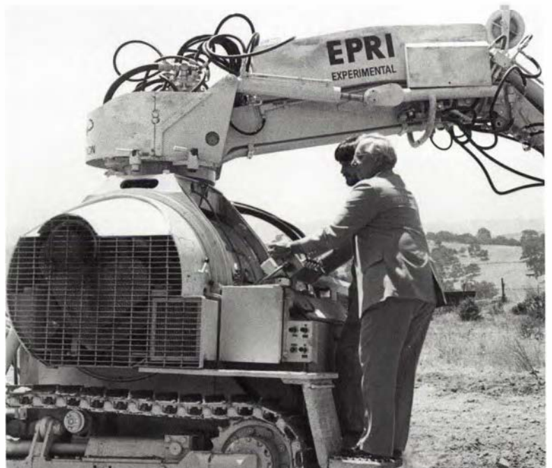
Culler at controls of prototype cable plow
