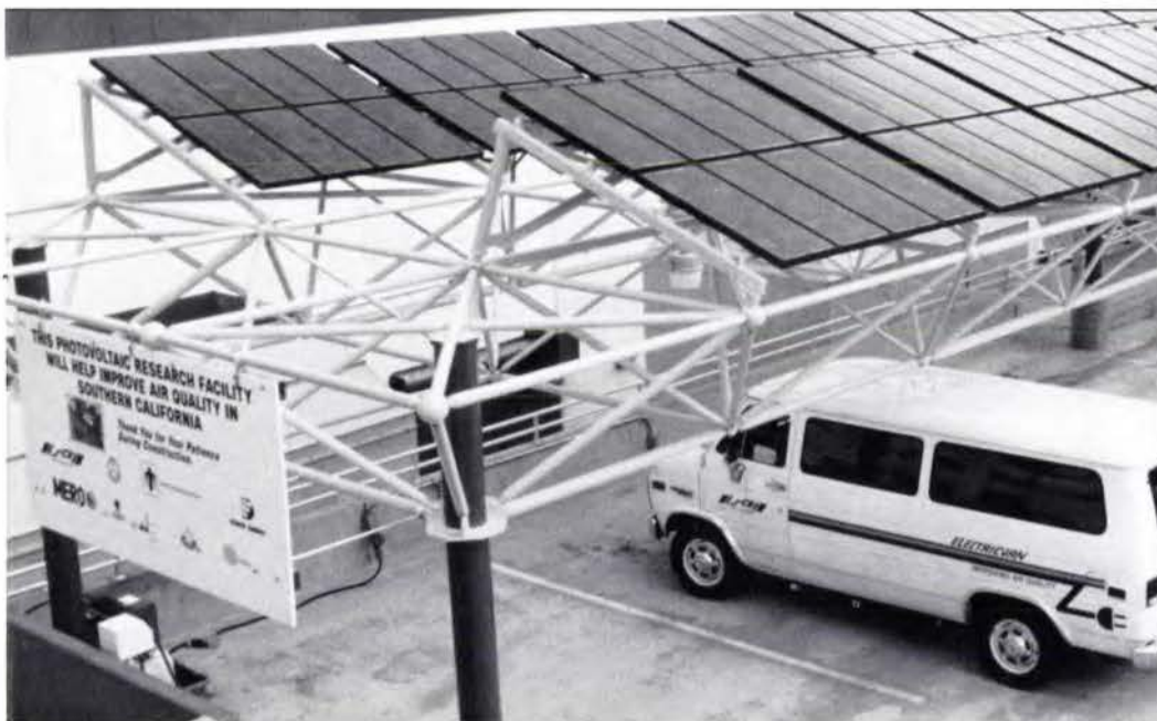
The solar-powered chargeport at the South Coast Air Quality Management District's office was a joint effort with Southern California Edison.
