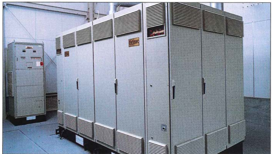
Two Westinghouse 20-kW units at the Rokka Island Test Center for Advanced Energy Systems (near Kobe, Japan), operated by the Kansai Electric Power Company. One of the units has run in excess of 6500 hours.
