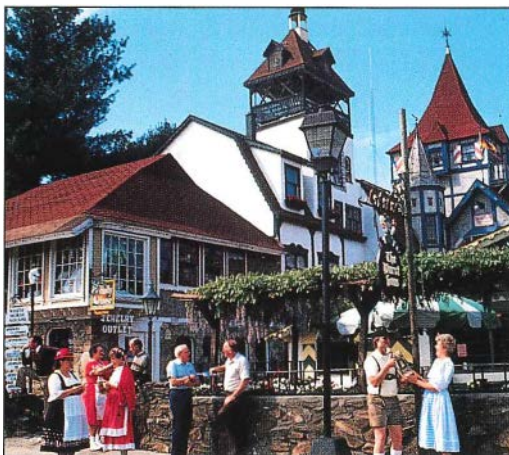
The Bavarian-style village of Helen, Georgia, draws thousands of tourists during its annual Oktoberfest celebration. The impending event put extra pressure on workers installing a 115-kV transmission line beneath the Nacoochee Valley floor last year. The workers regularly put in 14-hour days, finishing the job just two weeks before the festivities began.
