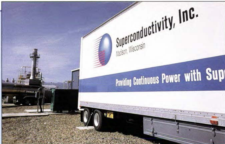
Trailer installation at CYANCO plant, Winnemucca, Nevada
