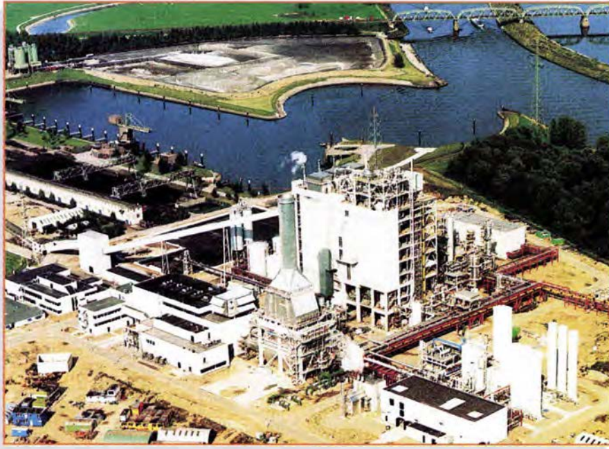
253-MW coal-fired IGCC unit now operating in Buggenum, Netherlands
