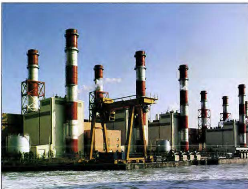
STATE-OF-THE-ART POWER PLANTS IN THE PACIFIC RIM Today's market-leading combined-cycle power plant designs are exemplified by Korea Electric Power Corporation's 1910-MW Seoinchon plant. The plant is currently composed of eight General Electric combined-cycle units, each of which includes a GE 7F gas turbine-generator and a reheat steam turbine-generator. The utility has undertaken a 2000-MW expansion at the plant and has selected GE to provide equipment and services. The additional combined-cycle capacity is expected to come on-line in 1997. (Photo: GE Power Systems)
