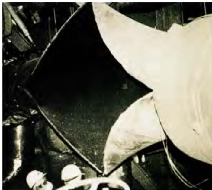
Figure 1 In power plants, the failure of seam-welded hot reheat piping, which carries steam at around 1000°F and 400–700 psig, is costly and potentially hazardous. Responding to catastrophic ruptures at two fossil plants in 1985 and 1986, EPRI developed the utility industry's only guidelines for evaluating the integrity and preventing the failure of such piping.
