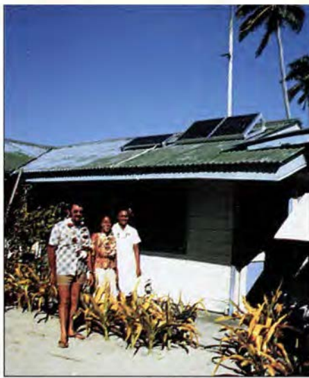
Rooftop photovoltaics at a medical center in Western Samoa.
