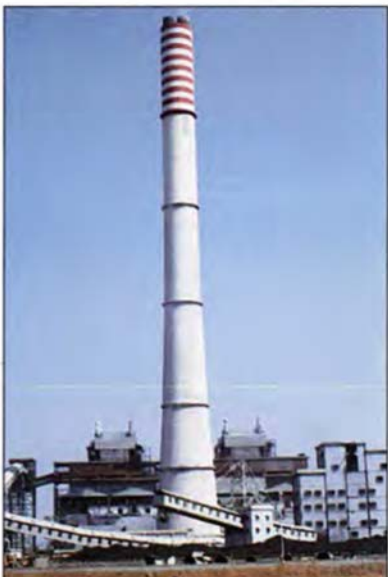
This two-unit, 500-MW coal-fired power plant at Dahanu, Maharashtra, began operating this year.
