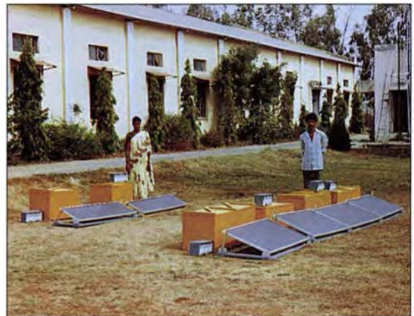
Charging battery-powered village lanterns with solar photovoltaics.
