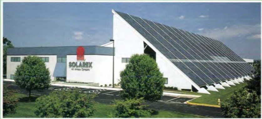
This Solarex building in Frederick, Maryland, now doubles as the headquarters for the joint venture Amoco/Enron Solar.
