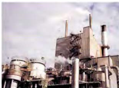
In Mobile, Alabama, Southern Electric International (a Southern Company subsidiary) purchased a 100-MW cogeneration unit that burns wood waste, coal, and crop residues from the former owner, Scott Paper; steam from the plant is sold to Kimberly-Clark, which recently acquired Scott Paper.
