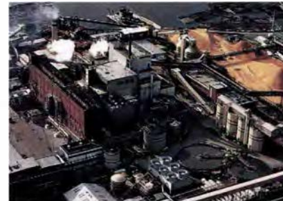
In Washington state, the Snohomish County Public Utility District provided the capital for a 38-MW cogeneration unit at Kimberly-Clark Corporation's Everett paper plant. The unit burns wood waste from area lumber mills, producing steam for Kimberly-Clark and electricity for the utility.
