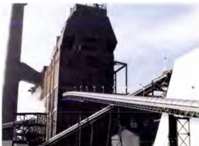
In the mid-1980s, Minnesota Power converted two 30-MW oil-fired units at its Mibbard plant in Duluth to fire mainly mill wastes to raise steam that is sold to a paper plant adjacent to the site. The utility is considering resuming power generation at one of the units.
