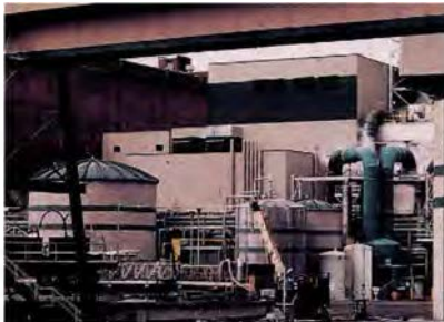
In Washington state, the Snohomish County Public Utility District provided the capital for a 38-MW cogeneration unit at Kimberly-Clark Corporation's Everett paper plant. The unit burns wood waste from area lumber mills, producing steam for Kimberly-Clark and electricity for the utility.
