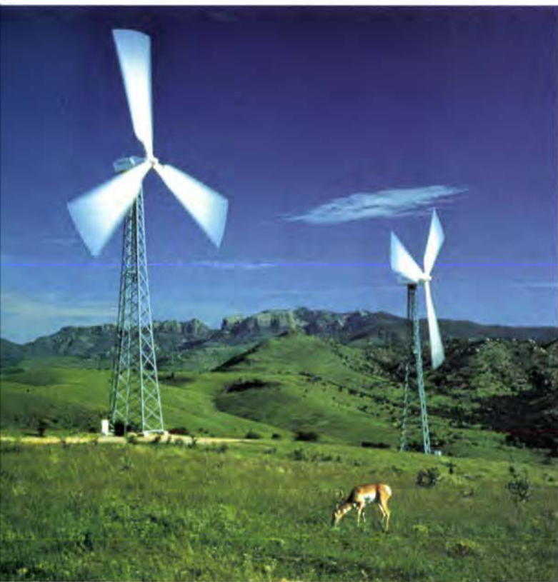
Electric utilities are deploying smaller clusters of wind machines. Shown here are two 500-kW turbines from a 12-unit wind farm in the service territory of West Texas Utilities.
