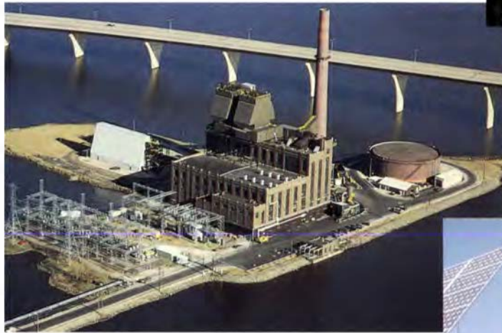
Wisconsin Electric customers voluntarily increased their monthly bills to put idle capacity of this biomass plant to use. The plant is fueled by waste wood from forest-product industries—scrap that would otherwise be trucked to a landfill.
