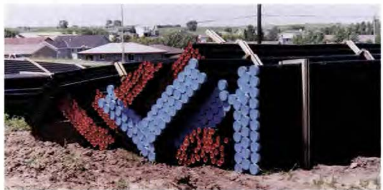
Heat pump system piping ready for installation
