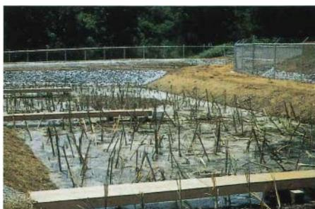
**Intelligent design and engineering of constructed wetlands are the keys to cost-effective cleansing of utility wastewaters. The constructed wetland at Allegheny Power's closed ash management facility near Springdale, Pennsylvania, includes four vegetated aerobic cells. To create these cells, basins were excavated and lined, substrates were installed, and various species of aquatic vegetation were planted.**
