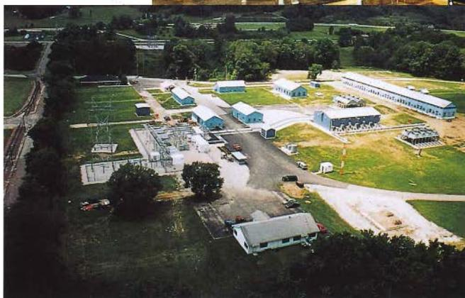
**COMPRESSOR UPGRADE LEADS TO ELECTRIC DRIVES** El Paso Energy's Catlettsburg, Kentucky, main-line compressor station upgraded over 14,000 hp of aging gas-fired compressor equipment with three electric compressor packages like the one shown here. Equipped with synchronous adjustable-speed drives, these electric units have reduced station maintenance costs and personnel requirements and have cut emissions of nitrogen oxides.
