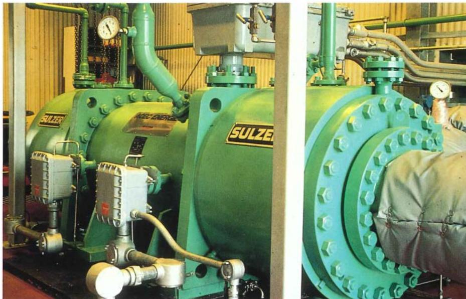
**TRANSCO DEMONSTRATES INTEGRAL UNIT** Transcontinental Gas Pipe Line Corporation installed an 8000-hp integral electric motor-compressor with an adjustable-speed drive at an Alabama compressor station to improve operating flexibility, reduce capital and maintenance costs, and lower emissions and noise levels. The ASD enables the unit to maintain high efficiency under all load conditions.
