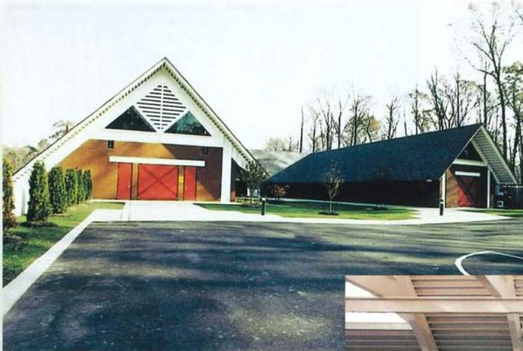
**Columbia Gas Transmission Corporation built its Rutledge compressor station in Maryland to conform to the architectural standards of the surrounding residential development. The company installed three integral electric motor-compressor units that don't disturb the neighbors or the environment.**
