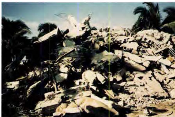
The 12-story Costa Real Hotel, located just north of Manzanillo, collapsed during the earthquake on October 9, 1995, killing 40 people.
