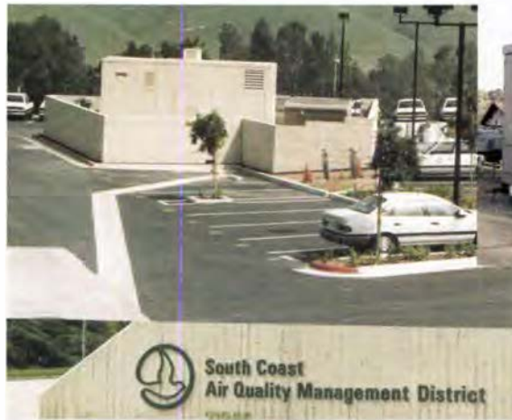
California installation of ONSI's 200-kW PAFC
