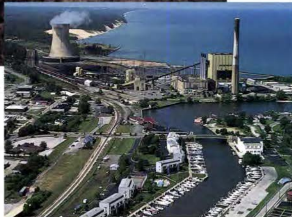
The Michigan City generating station—a 500-MW coal-fired plant bordered by a mall, a marina, and a national park—was selected by Northern Indiana Public Service Company as the first of its facilities to adopt ISO 14001. It became the first U.S. coal-fired plant to be registered to the new standards.
