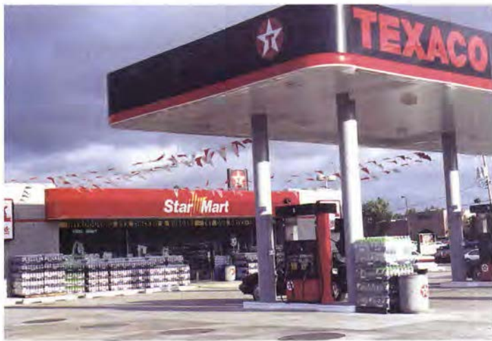
Equipped with a geothermal heat pump system for heating, cooling, and refrigeration, this Texaco Star Mart station in Oklahoma City uses 27% less energy than a comparable station 5 miles away that has conventional equipment.
