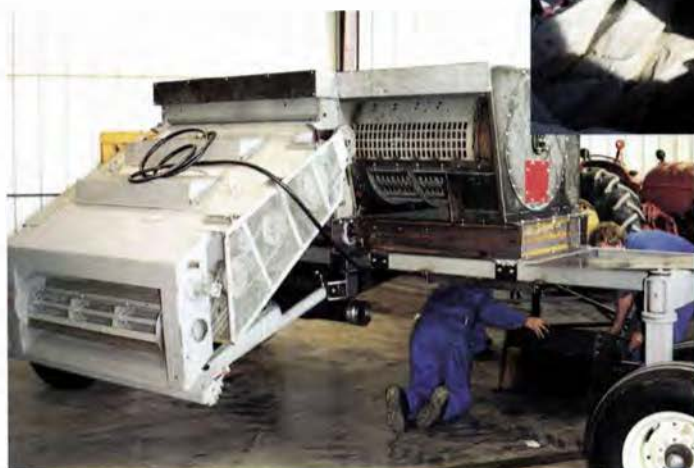
Mobile field unit under construction
