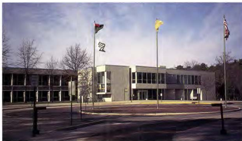
Richard Stockton College in Pomona, New Jersey, is home to what is believed to be the world's largest single closed-loop piping network, which provides a cooling capacity of 1600 tons.
