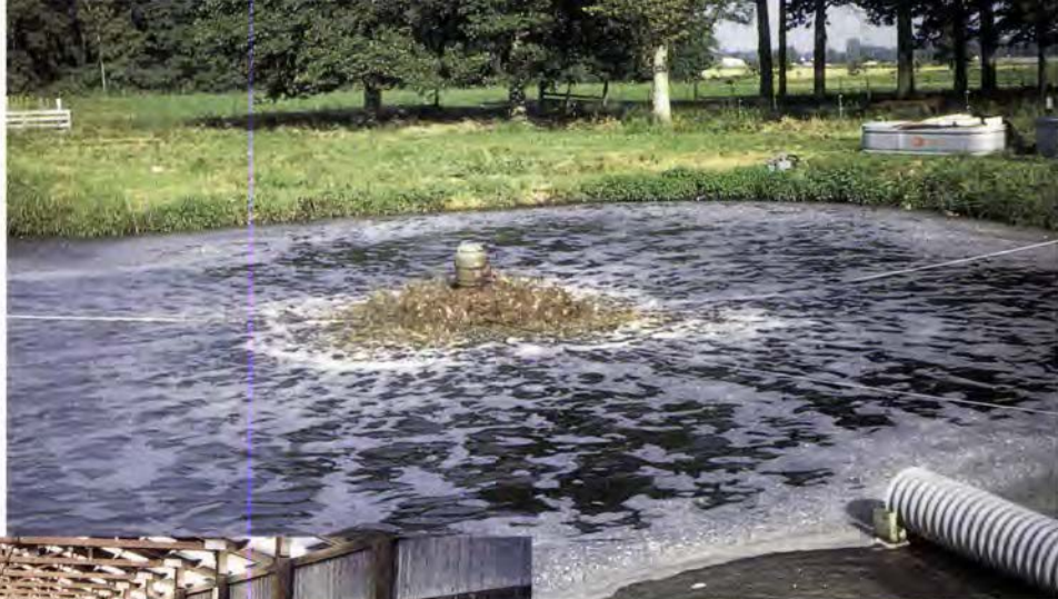
Wastewater pool with aerator
