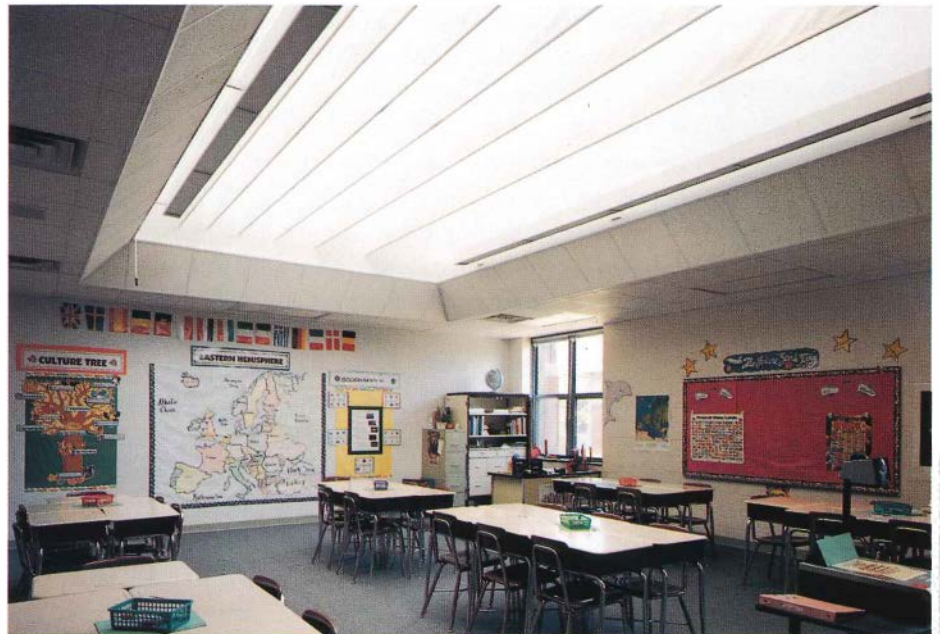
Several elementary schools near Raleigh, North Carolina, reported improved achievement test scores among students who moved into daylit classrooms. This classroom features a roof monitor-type skylight with light-diffusing baffles.
