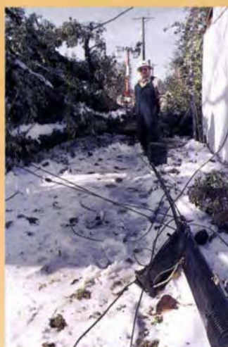
A distribution line felled by a severe snowstorm in OPPD's service territory
