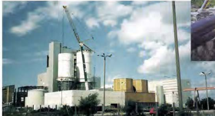
This CHP plant in Cottbus, Germany, will use pressurized fluidized-bed technology to burn local brown coal. It is scheduled to be on line by mid-1999 and to eventually replace an old, polluting coal-fired plant.
