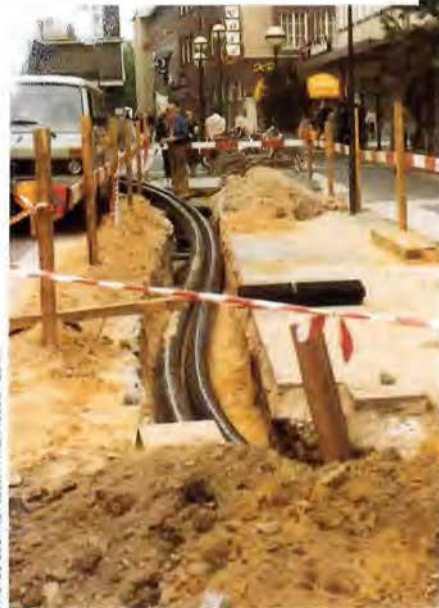
Flexible hot water piping being installed in Germany
