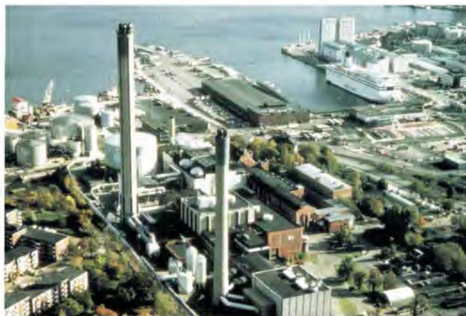
Stockholm Energi's Värtan CHP plant has two pressurized fluidized-bed combustion units that burn low sulfur coal.
