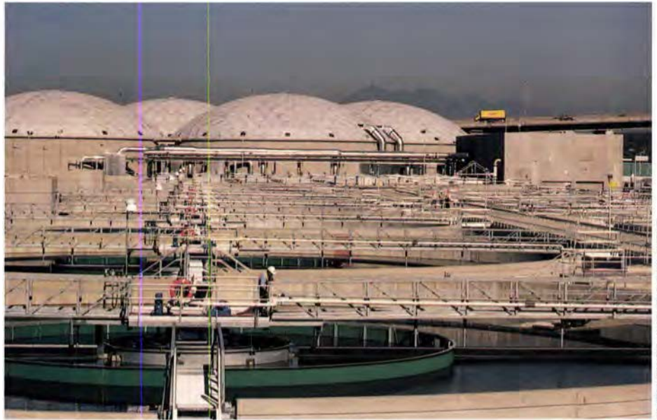
Annacis Island wastewater treatment plant, Vancouver
