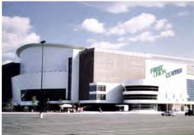
A new controller for optimizing ice storage systems was successfully tested at this Philadelphia arena.
