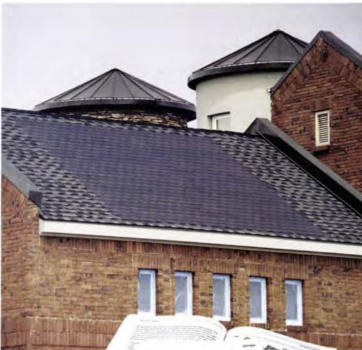
COURTESY UNITED SOLAR SYSTEMS CORP.
