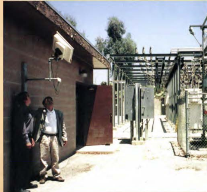
Southern California Edison uses its Ultra-Net system to monitor and control over 150 remote substations in its service area. Ultra-Net features very small antenna (0.3-meter), flat-array ground terminals, which communicate with a GEO satellite via Ku-band microwave.
