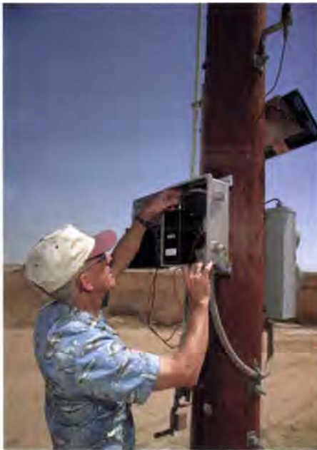
As a value-added reseller of Orbcomm USA services, Salt River Project markets Spatia—a satellite-based system for near-real-time communications and the processing of remote monitoring and metering data for water, electricity, and natural gas utilities in the western states.
