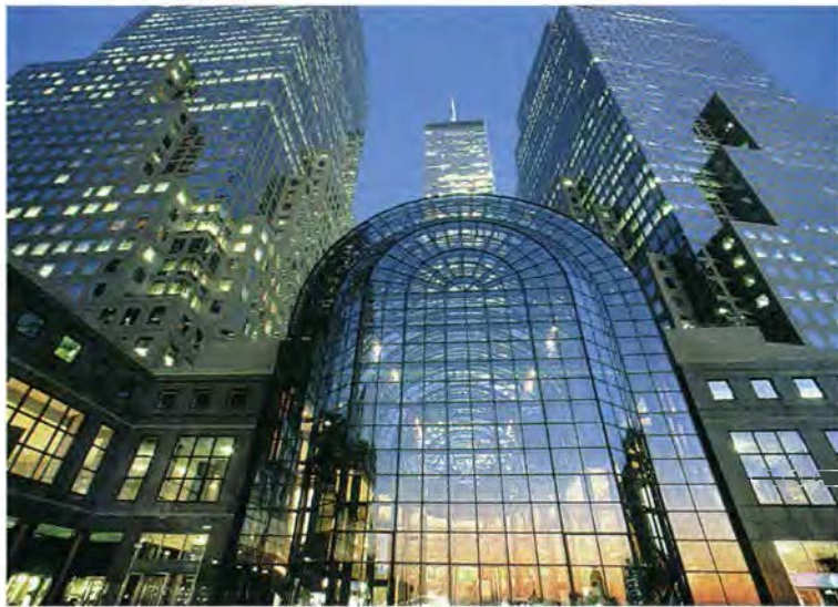
The New York Power Authority called on EPRI/PEAC Corporation for assistance with an intractable lighting problem at a high-profile customer site: the lobby of the World Trade Center's twin-tower office complex. By simulating the lobby's lighting setup and operating environment in the laboratory, PEAC was able to pinpoint the source of the problem and develop an inexpensive solution without disrupting business operations at the center.
