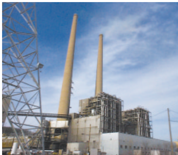
COURTESY AMERICAN ELECTRIC POWER
