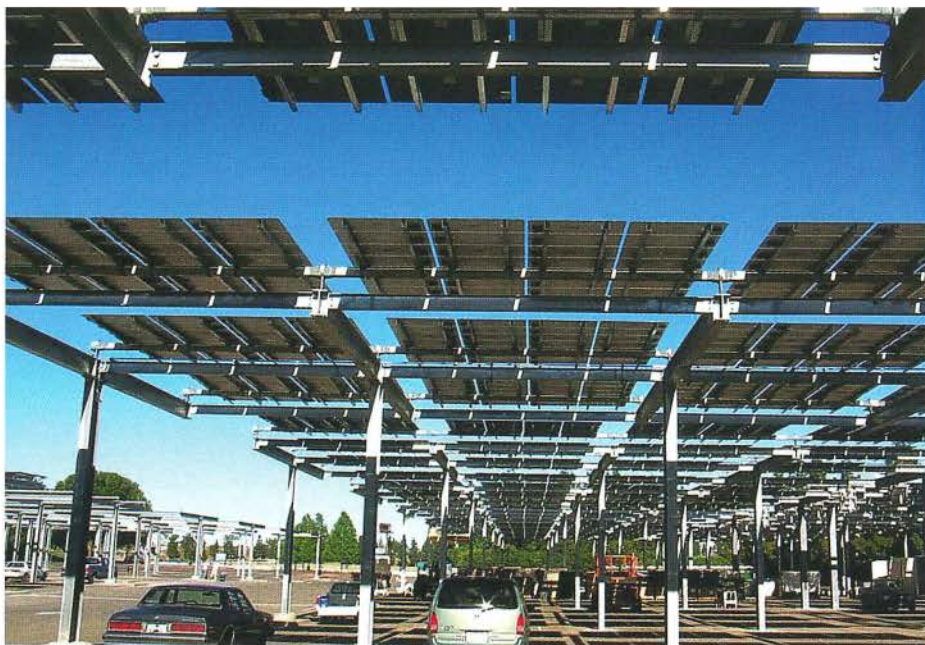
The Sacramento Municipal Utility District has installed a 540-kW PV system in a parking lot at Cal Expo, site of the California State Fair. The sun-tracking arrays, made up of 13,700 PV modules, provide shaded parking for more than 1000 cars.
