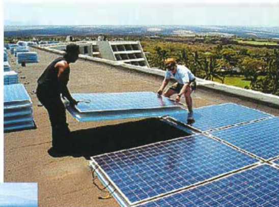
A 73.6-kW (ac) system using ASE Americas PV modules, installed for the Hawaiian Electric Light Company by PowerLight Corporation on the Mauna Lani Hotel on the Kona coast of Hawaii.
