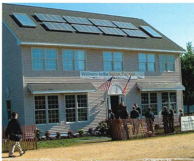
This 100%-solar-powered modular home, featuring both rooftop and building-integrated PV technologies, was erected on the National Mall in Washington, DC for the American Solar Energy Society's annual meeting in April 2001.
