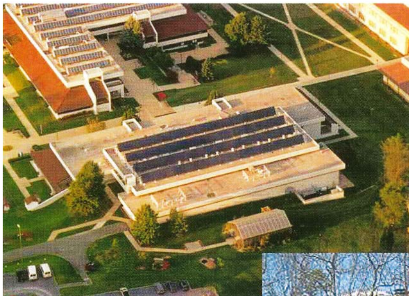
A 2.9-kW (ac) system using Solarex PV modules is installed on Montgomery County Community College in Germantown, Maryland.
