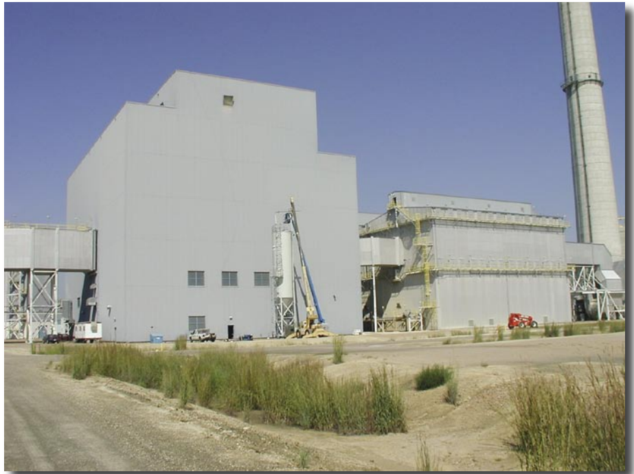
Sunflower Electric's Holcomb Station near Garden City, Kansas, was host to a full-scale field test of sorbent injection for mercury capture under the DOE-NETL program. Conventional sorbents injected into the flue gas duct (far left) before the plant's spray dryer unit achieved only modest results in removing mercury. However, use of a new, chemically enhanced sorbent removed 90% of the mercury at low-to-moderate injection rates. The sorbent is collected by the plant's fabric filter, and the cleaned flue gas exits the stack at right. (Photo courtesy ADA-ES)
