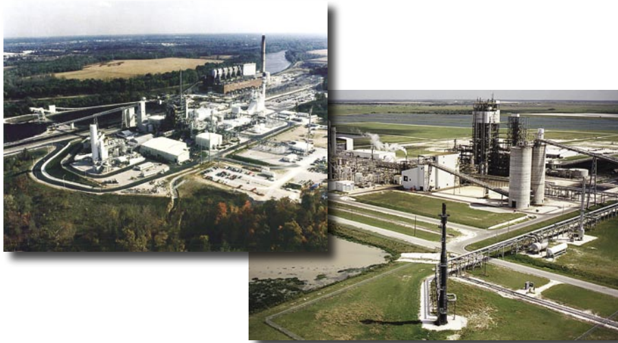
Two demonstration projects supported by DOE and the industry have paved the way for the deployment of IGCC technology. Cinergy was host to a 262-MW IGCC repowering demonstration at its Wabash River Generating Station near Terra Haute, Indiana, in 1995. Tampa Electric's 250-MW Polk County IGCC demo is a green-field unit that began operation in 1996.
