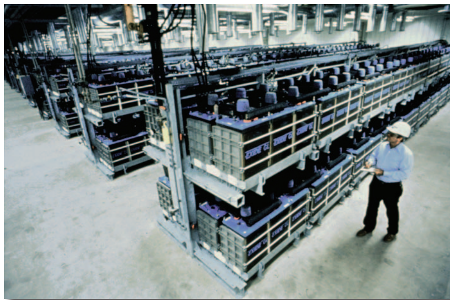
Large-scale battery storage was demonstrated in the mid-1980s at Southern California Edison's Chino facility, which offered 10 MW of power with a 4-hour discharge capability using lead-acid batteries. Such projects paved the way for more-advanced battery projects, including a recently built 27-MW, 15-minute-discharge nickel-cadmium installation in Fairbanks, Alaska.
