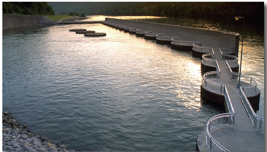
Pumped-hydro facilities such as TVA's 1.6-GW Raccoon Mountain plant represent the most mature option for large-scale utility applications like daily load shifting. There are currently 150 such U.S. facilities operating in 19 states; however, high construction costs and a scarcity of suitable surface topography are likely to severely limit further development of pumped-hydro storage in this country.
