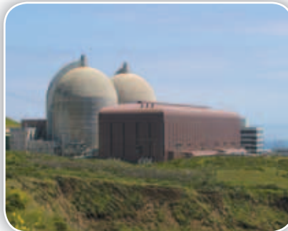
Diablo Canyon Nuclear Power Plant, just west of San Luis Obispo, California (Photo courtesy Jim Zimmerlin.)
