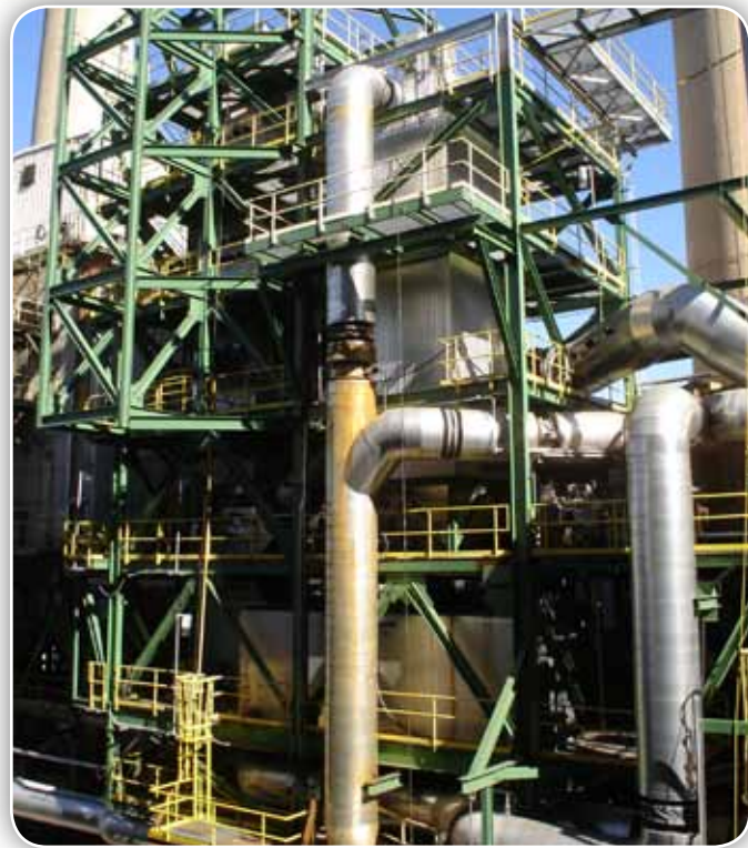
Gulf Power's Mercury Research Center
