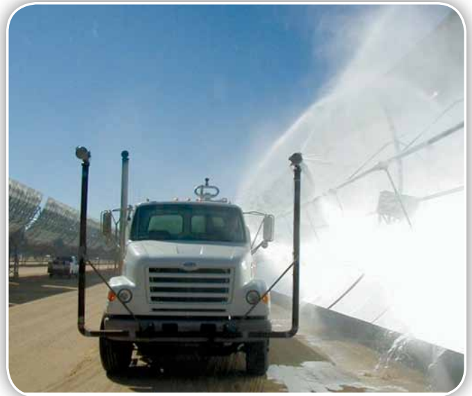
Mirrored collectors at solar thermal plants must be washed as often as once a week.
