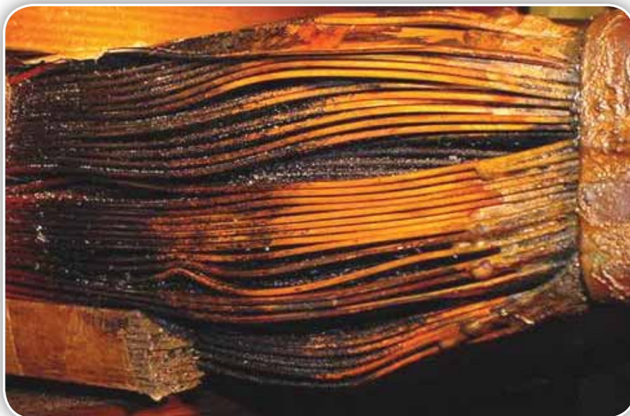
Geomagnetically induced currents can saturate transformers, causing them to demand high levels of reactive support, produce large amounts of harmonics, and generate heat that can damage high-voltage and generator step-up transformers.
