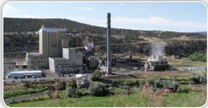
Tri-State's 100-MW Nucla Station
