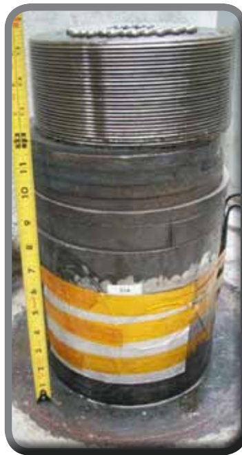
Fiber-optic strain gauge installed on a tendon anchor
