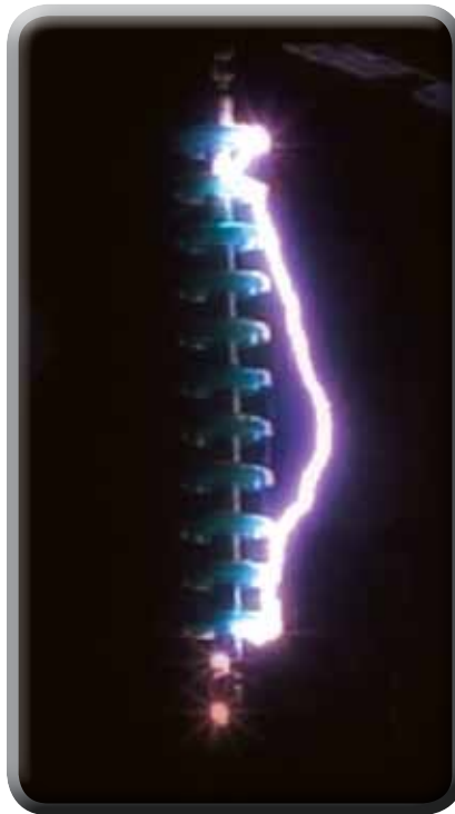
Flashover with two broken discs at the live end
