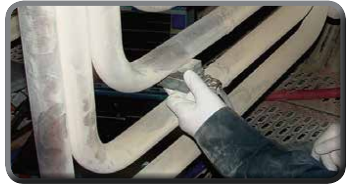
Portable electromagnetic scanner checks boiler tubes for magnetite
