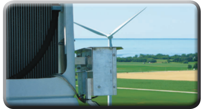
Ultrasonic microphones coupled with sophisticated modeling software allow wind turbines to be automatically shut down when bat activity is detected.
