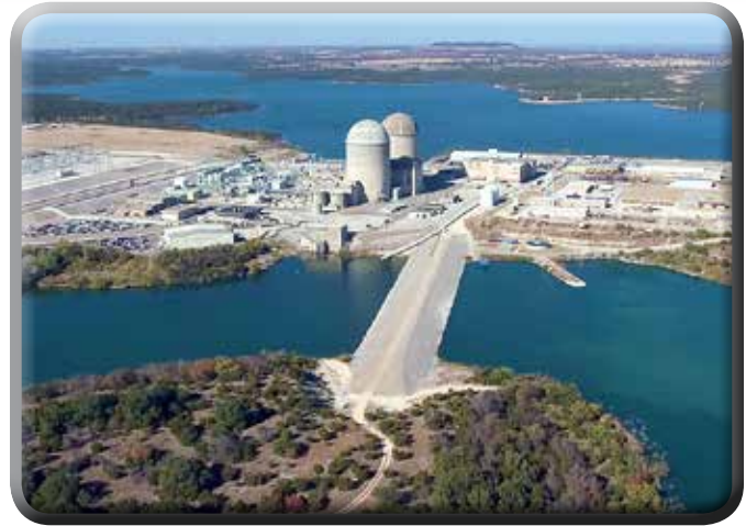
Comanche Peak Nuclear Power Plant Source: U.S. Nuclear Regulatory Commission
