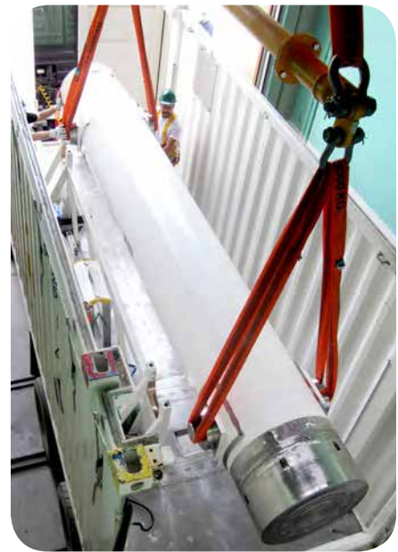
The cask with irradiated materials is lifted out of the fuel pool (left) and then loaded into the container (right).
