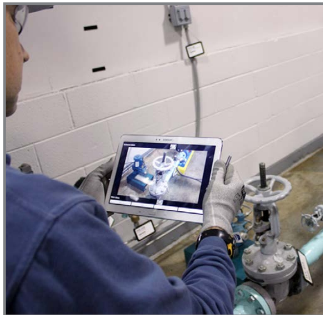
A plant technician uses the tablet technology to verify the completion of a valve alignment.
