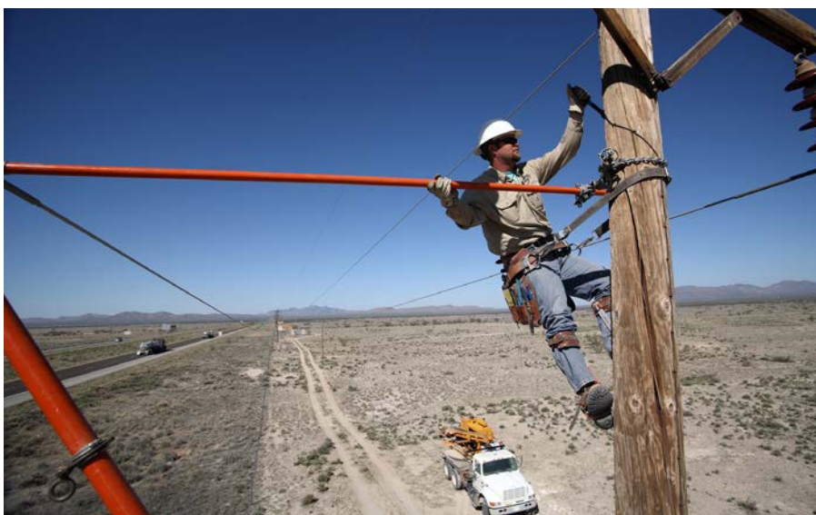
A line worker using a hotstick. Photo courtesy of NRECA.
