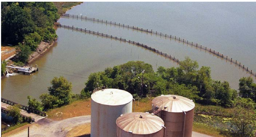
A barrier net at NRG's Chalk Point Power Station in Maryland
