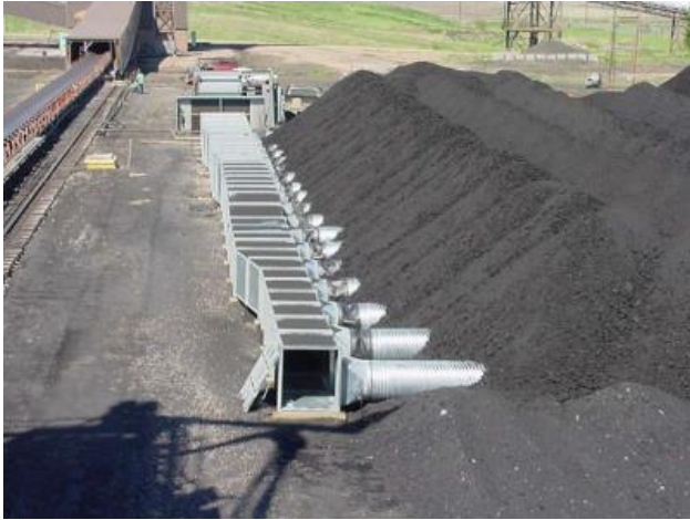
Concept: In 1997, Great River Energy used propane heaters and an old culvert to experiment with the lignite-drying process.
