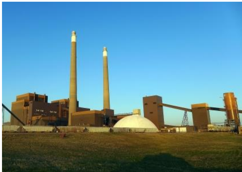
Coal Creek Station’s power plant (the brown building on the left) houses the commercial-scale DryFining facility.
