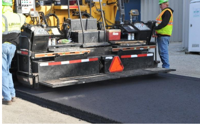
Ease of use: The introduction of fly ash to asphalt didn't require any new equipment or change in process for the crews that paved the road at the Oak Creek coal plant.
