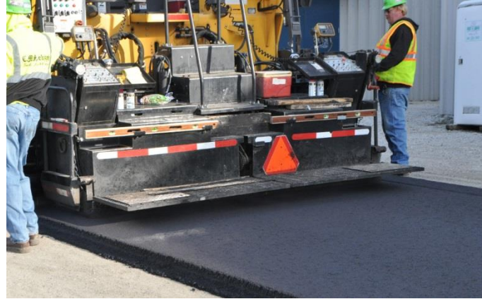
Ease of use: The introduction of fly ash to asphalt didn't require any new equipment or change in process for the crews that paved the road at the Oak Creek coal plant.
