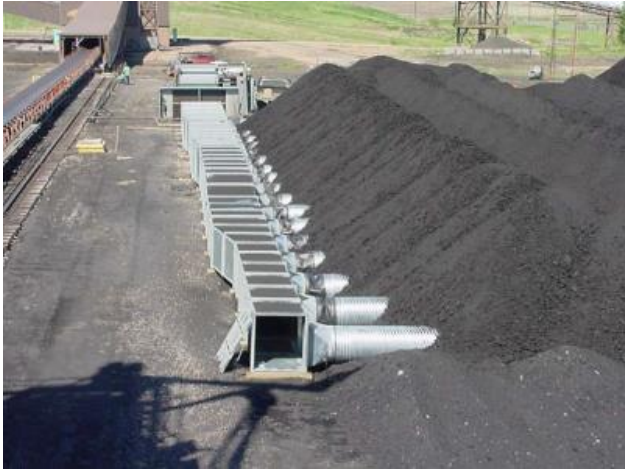
Concept: In 1997, Great River Energy used propane heaters and an old culvert to experiment with the lignite-drying process.
