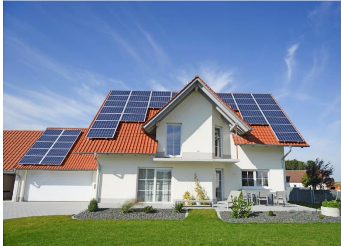
DERMS are new types of software and communication systems that manage distributed energy resources such as solar photovoltaic systems.
