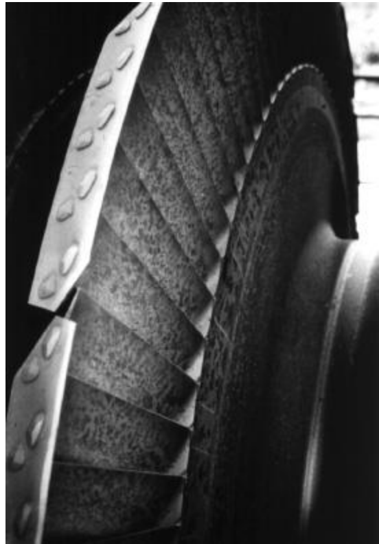
Corrosion on a turbine
