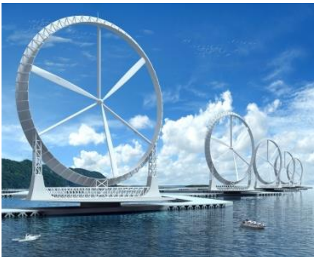
Image Provided by Prof. T. Ohta, Kyushu University The Research Institute for Applied Mechanics at Japan's Kyushu University uses a distinctive wind lens to draw more wind into offshore turbines. In this concept, multiple turbines can be deployed on floating platforms rather than seabed-mounted towers. Note that this image is synthetic.
