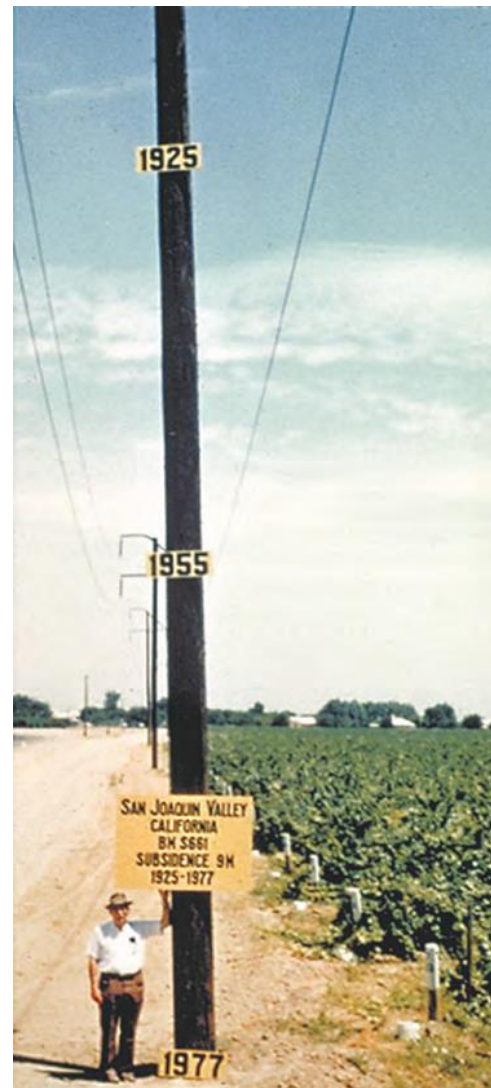
Subsidence largely due to groundwater withdrawals in California's San Joaquin Valley
