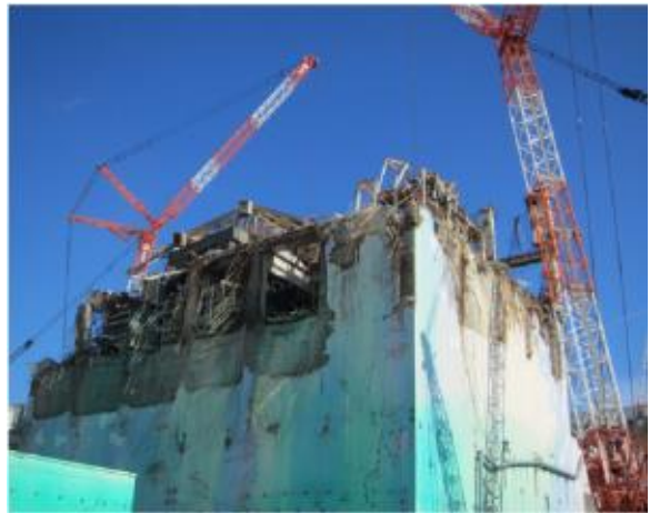
Clean-up of rubble at Fukushima Unit No. 3 in preparation for future fuel debris removal
