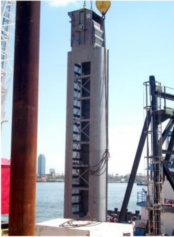
Con Edison installs the first of five new fish protection—modified traveling water screens at its East River Generating Station in 2012.
