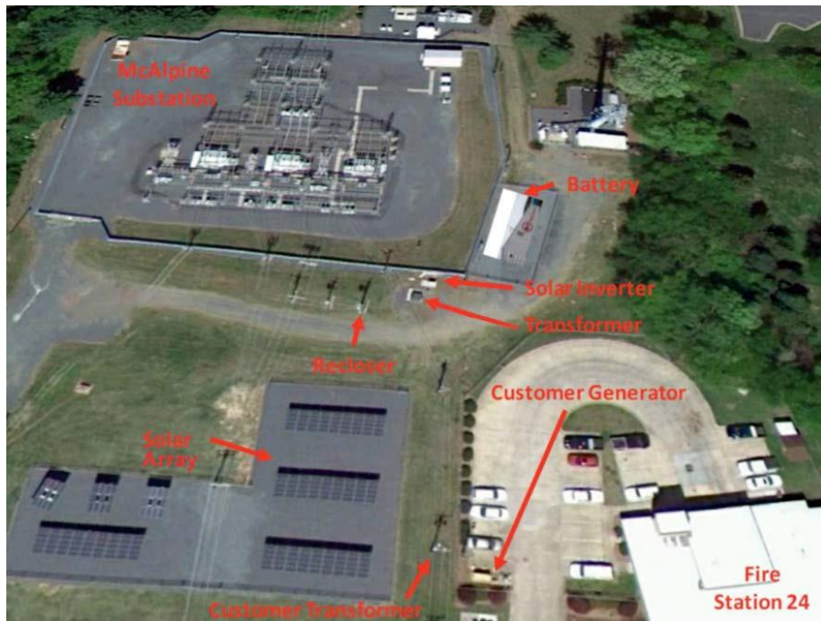
A microgrid in Duke Energy's service territory
